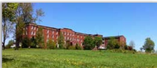
Bethany Motherhouse and the surrounding land before deconstruction
